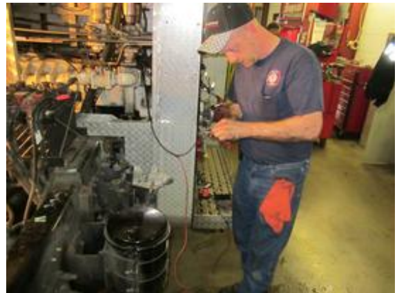
Finishing the wiring so that the primer control switch is powered when the pump is placed in pump gear.
