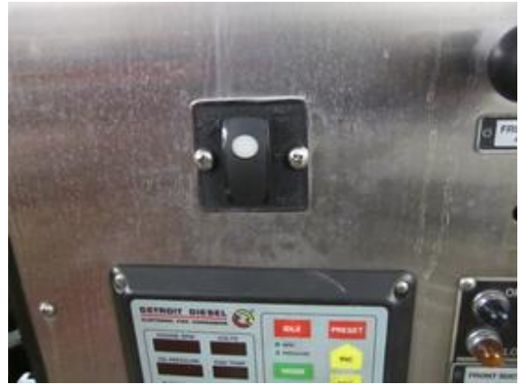
The new control switch is in place using the same hole that the old control handle used - just had to enlarge the hole a little bit.
