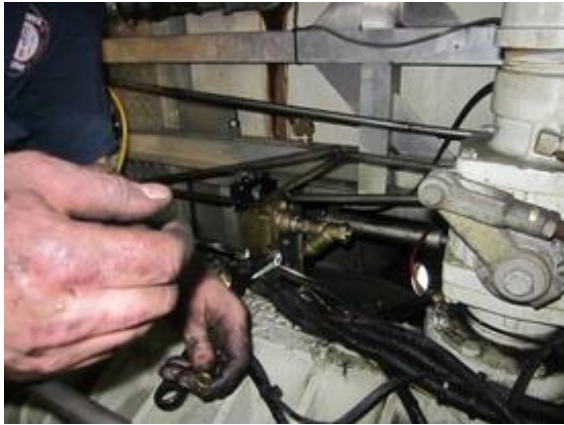
All in place - not is it time to run the control wires and air line.
