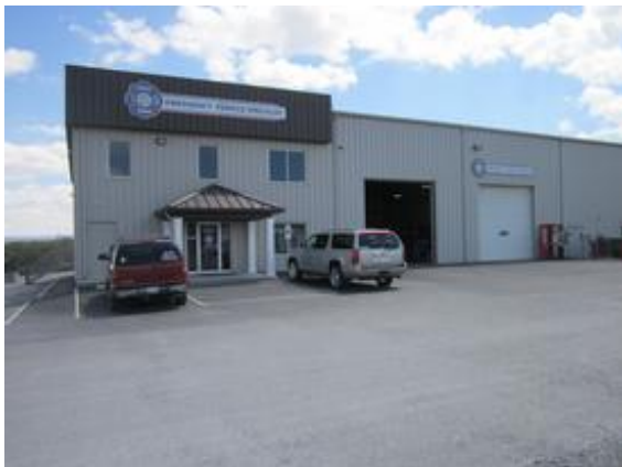
The air primer was installed by the folks at EVS in Hagerstown, MD.
