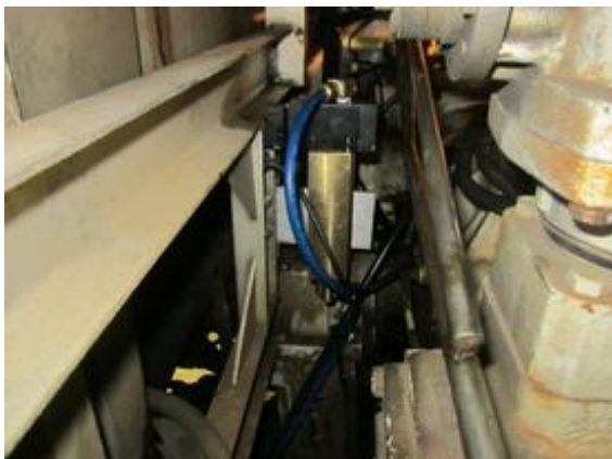
The air supply line (blue) is attached to the primer. The line receives its air from the pumper's air brake system.
